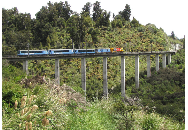
Overlander going over the new Hapuawhenua viaduct Photo: Roy Simons
