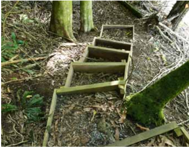
The steps are ready and waiting to be filled.
