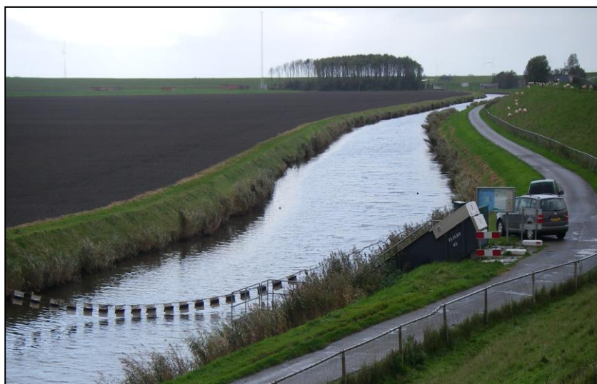
Figure 32: Light barrier in use in the Netherlands. The lights can be lowered into the canal by reducing the tension on the support cable. (photo – J. Boubée, NIWA)
