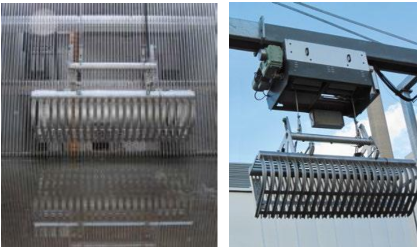
Figures: 14 – 16: (Top) Rotary screen cleaner Piripaua Power Station intake (Waikaremoana Power Scheme). (Bottom) Grab screen cleaner, Wairere Fall Power Station Mokau River. (Screen cleaner originally from Karapiro Dam) (photos J. Boubée, NIWA)
