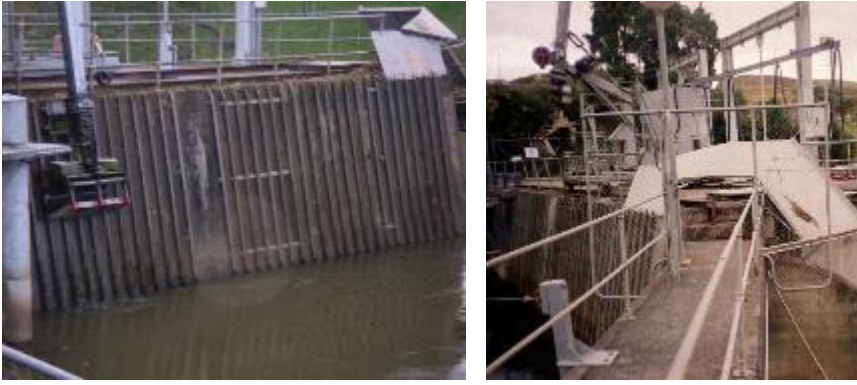
Figures: 14 – 16: (Top) Rotary screen cleaner Piripaua Power Station intake (Waikaremoana Power Scheme). (Bottom) Grab screen cleaner, Wairere Fall Power Station Mokau River. (Screen cleaner originally from Karapiro Dam) (photos J. Boubée, NIWA)
