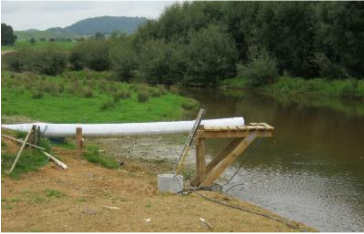
Figure 51. Projection of the fish ramp at Mokauiti Dam, King Country. The pipe passes through the stop bank above flood levels and allows fish to reach the open channel. For monitoring purposes or to transfer the catch further upstream it is possible to add a trap at the end of the ramp. (photo: J Boubée, NIWA).
