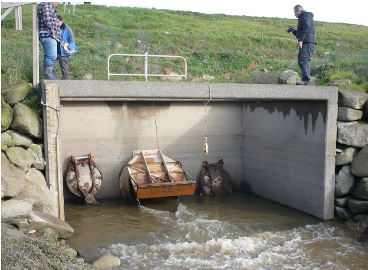
Figure 46. Flapgate winched to open position outside of flow periods to maximise opening for gravity flows and fish passage (photo: J. Boubée - Niwa)
