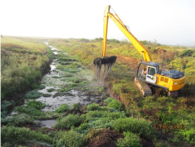
Figure 12: Prolific weed growth in drainage channel directly above pump station requiring mechanical removal (photo – WRC)
