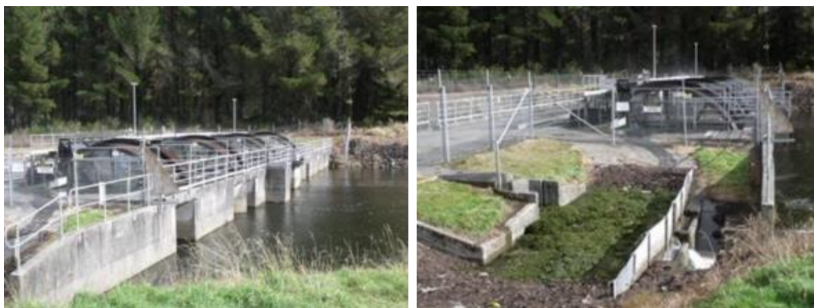
Figures 20 & 21: The Wairehu drum screen (Tongariro Power scheme) and weed collection point where trapped migrant eels are collected. (Photos: C. Speedy, Genesis).
