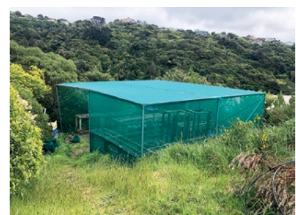
Work on the shadehouse #17 is now complete, the old framing covered in new cloth with new, more wind-resistant fixings.
