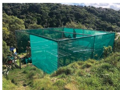
Work on the shadehouse #17 is now complete, the old framing covered in new cloth with new, more wind-resistant fixings.
