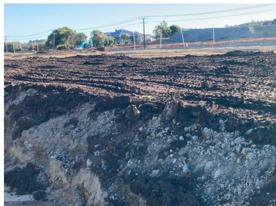
Peat laid on top of sand and clay base
